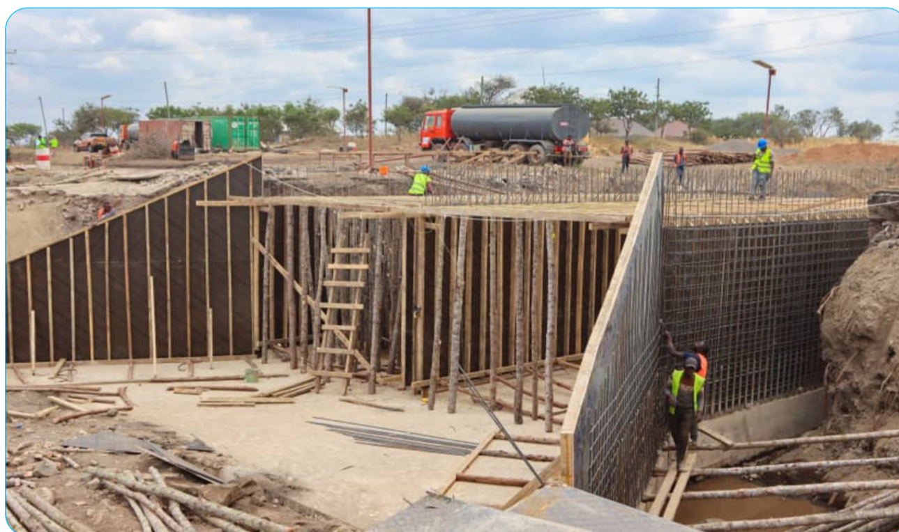
Biriri Bridge at Kwa Msomali in Hai, Kilimanjaro Region, under construction
